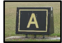
Taxiway Location Sign
