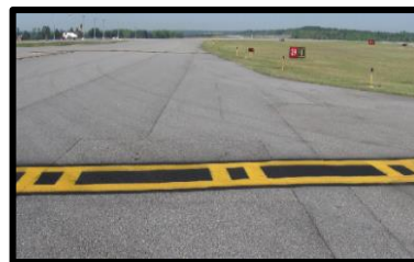
ILS Critical Area Boundary Marking
