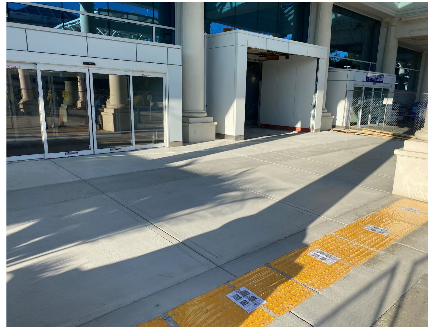
Terminal Front Water proofing, doors and pavement
